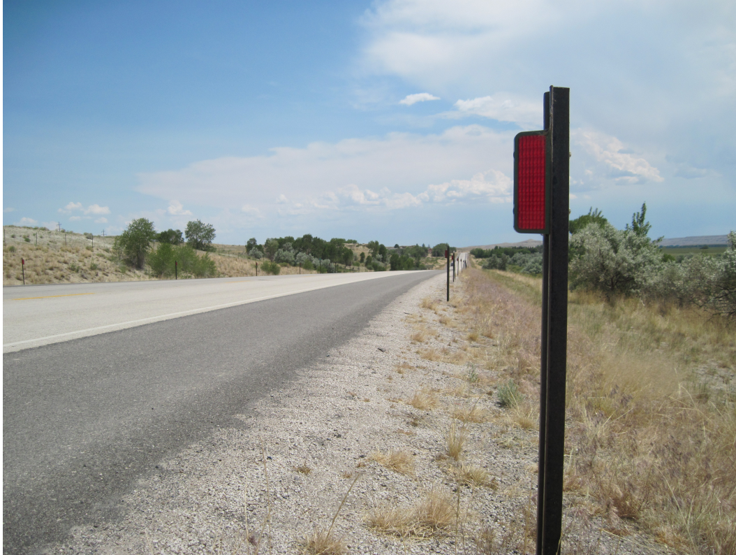
Figure 1. Wildlife warning reflectors installed along a stretch of highway.
